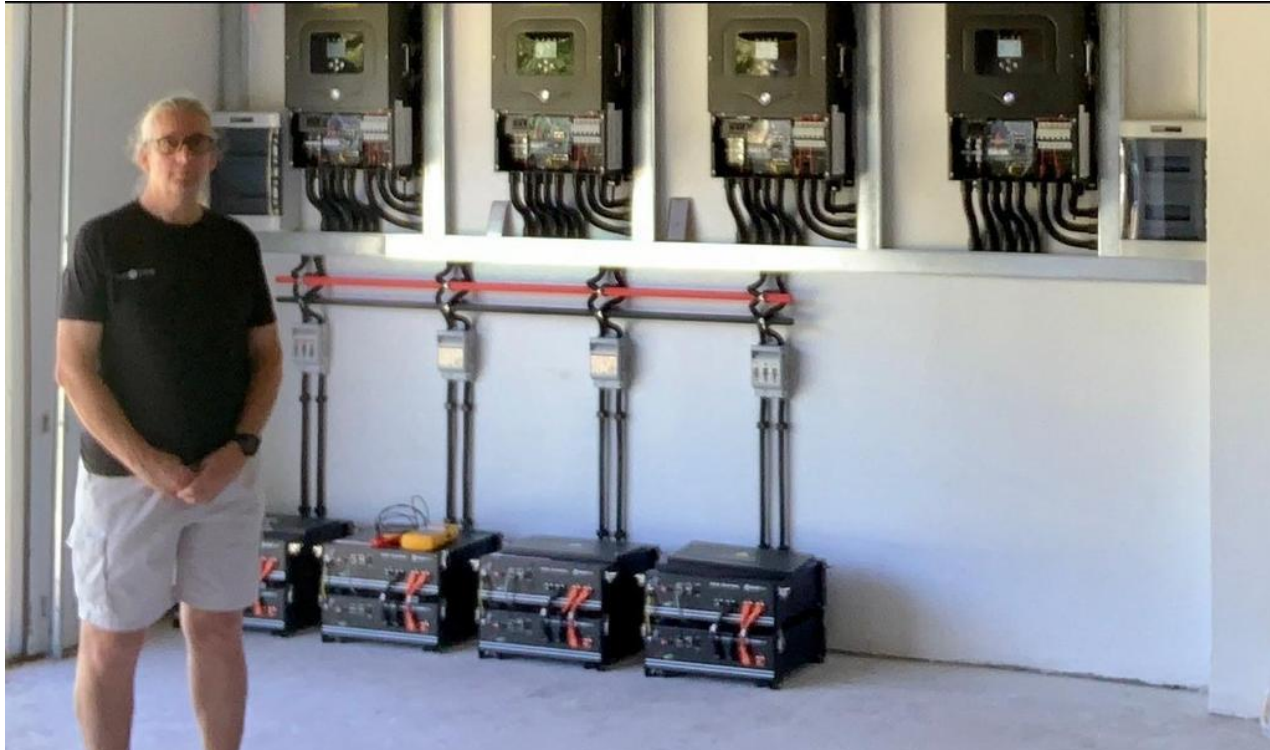
Figure 12 – Keith Gough at a Sunsynk installation in Port Elizabeth.
