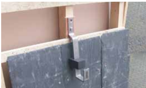
Step 1: Fix foam to bracket drop.
