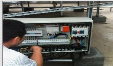
2、remove the PV string to be inspected
