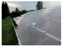
Horizontal mounting of laminated (thin-film) modules
