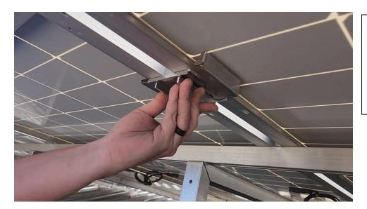
Place the Securi-link bracket underneath your panels, placing them between your panels in the 20mm gap.
