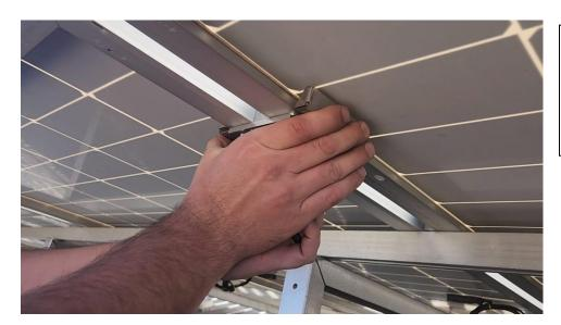
Squeeze the securilink bracket so that the stainless-steel lip slots over the lip of the panel frame.
