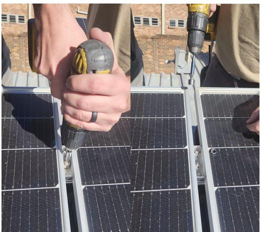
Tighten the 3 shear nuts on the top of the securi-link bracket between the panels until the shear nuts break loose.
