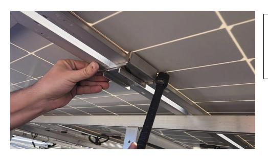
Gently tap the two slides on the securi-link bracket to make sure they are tight on the panel frame.
