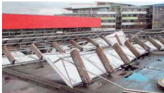
Example picture: Module rows damaged by overturning on a flat roof (insufficient loading) Source: Specialized press
