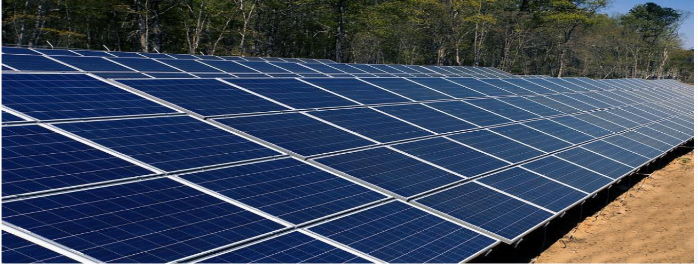
12.8MW Ground-mounted PV Plant in Melksham, UK
