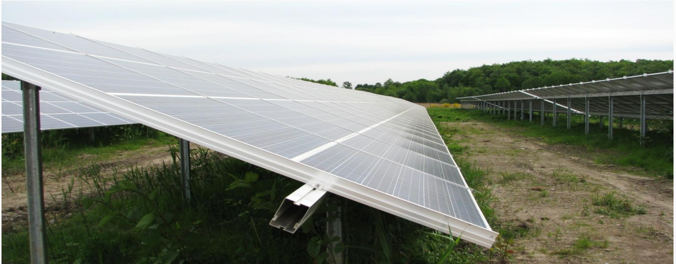
2MW Ground-mounted PV Plant in Guntramsdorf, Austria
