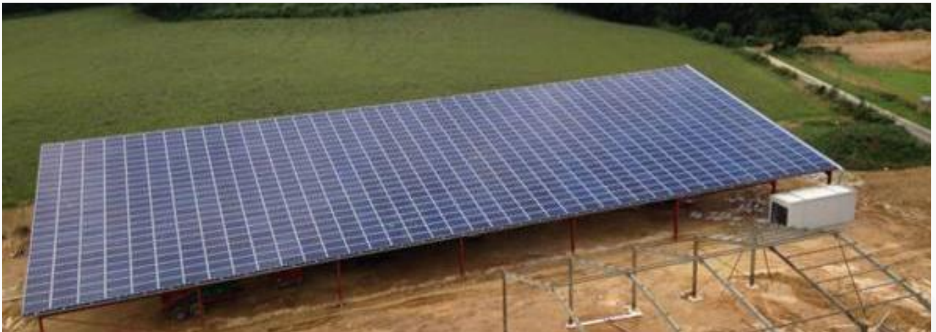
1.7MW Ground-mounted PV Plant in Friedland, Germany
