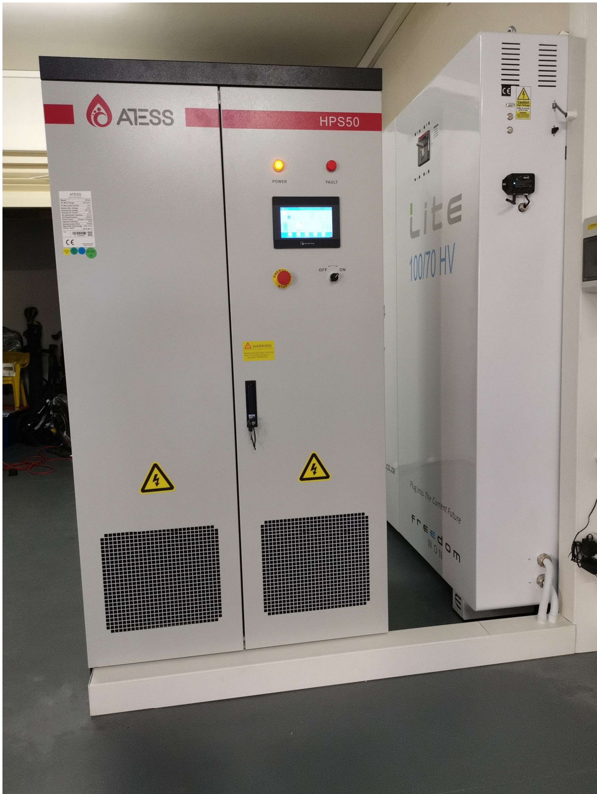
Fig 2.3 Installation Example of a Lite Commercial 100/70HV (now 100/80) with a ATESS HPS50 and no cable trench (trunking used instead)
