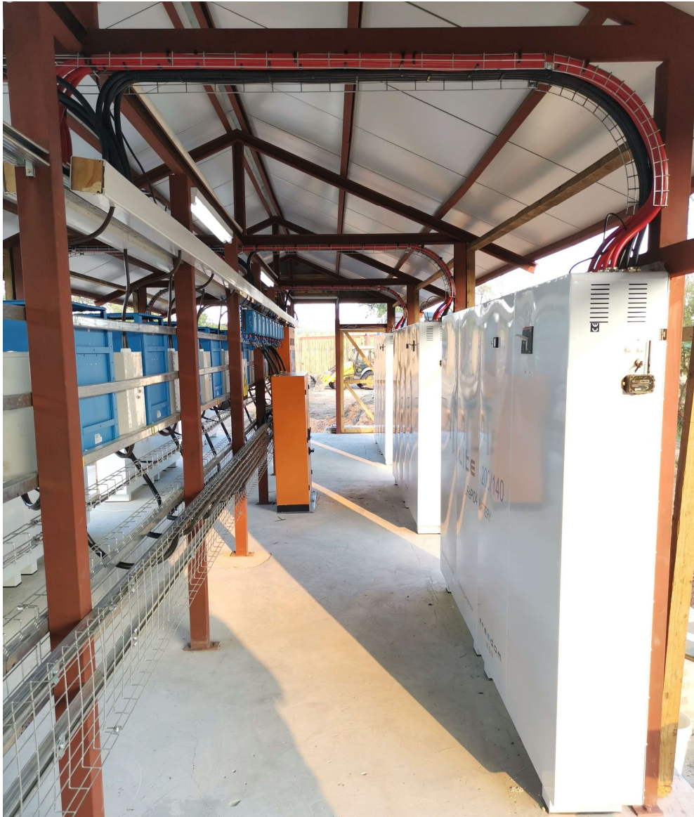
Fig 2.2 Top Cable Exit Example on a Lite Commercial 200/140
