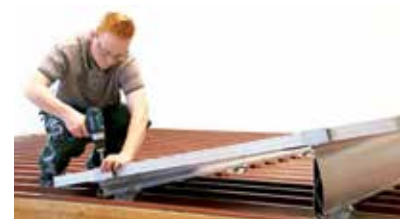
3 Mounting of the modules
