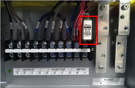
Critical components of BAT fuse
