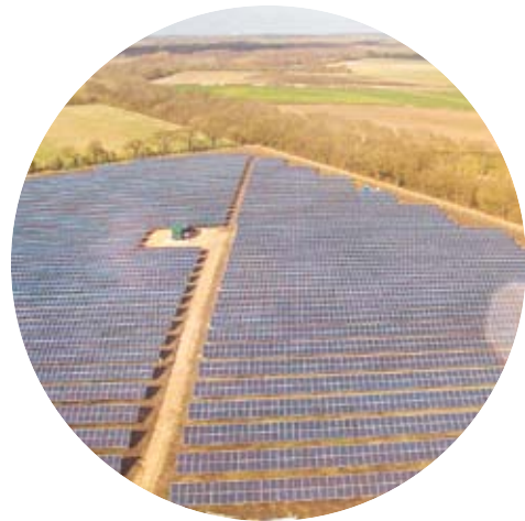
1. MOAT FARM, UK Module: CS6P-P Power generation: 4.61 MW
