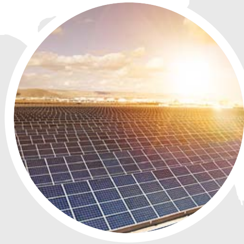
5. LARGEST ROOFTOP PROJECT, KAYSERI, TURKEY Module: CS6P-P Power generation: 2.3 MW
