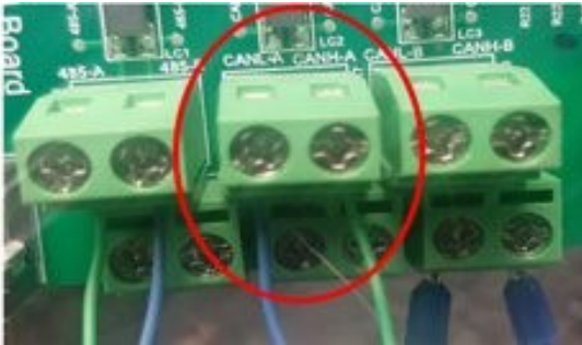
Figure 3: Inverter CAN pins for BMS communication.
