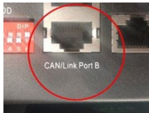
Figure 2: CAN port for BMS communication
