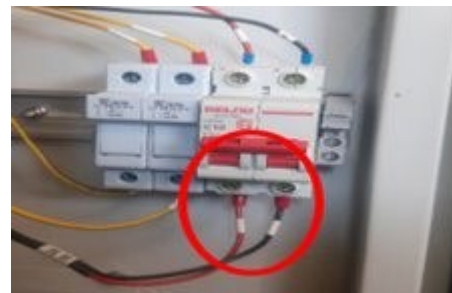
Figure 8: Control board DC power breaker on ATS.
