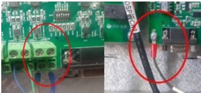
Figure 5: HPS CAN-B terminals and ground connection.
