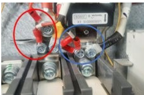
Figure 7: DC Power cable connections to ATS
