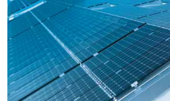
1. Photovoltaic modules on the roof generate sustainable energy for production facilities and office buildings.
